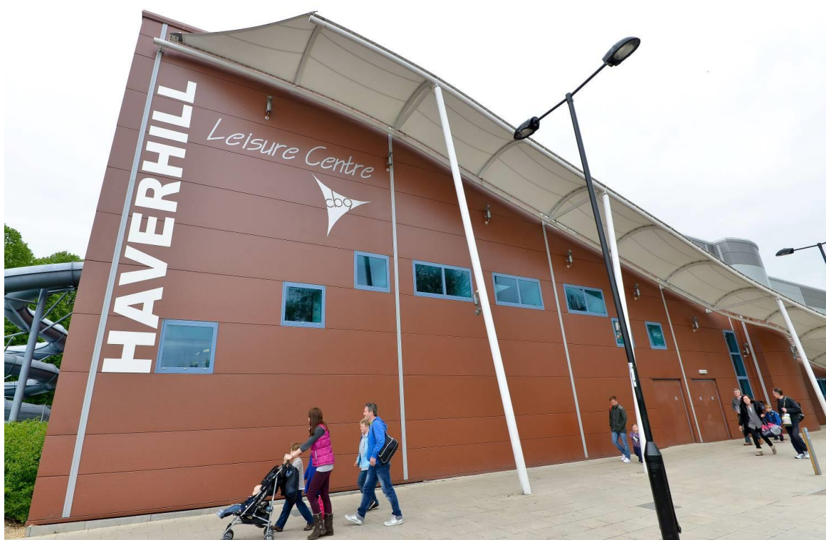
Haverhill Leisure Centre
